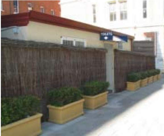
Public toilet entrances clearly visible from adjoining streets and squares for after hours surveillance.
