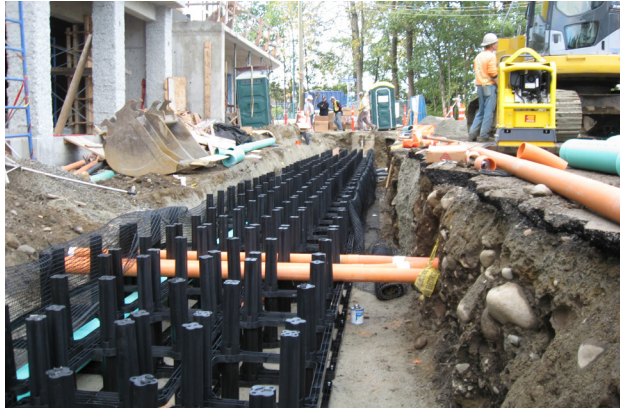
Underground services running through structural cells
