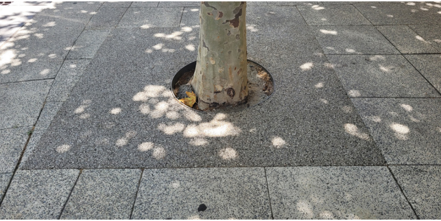
Porous resin bound aggregate (RBA) paving is the City’s preferred treatment to be retrofitted around established trees which have outgrown their grates or pits.
