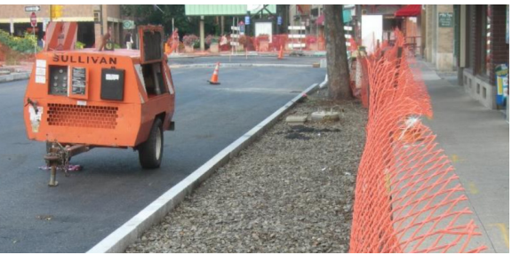
Structural soils support the pavement above, whilst providing quality soil for tree roots below
