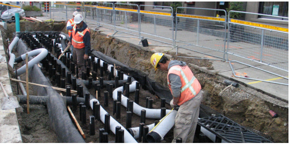
Structural cells can and should be installed around existing underground services and include water harvesting systems
