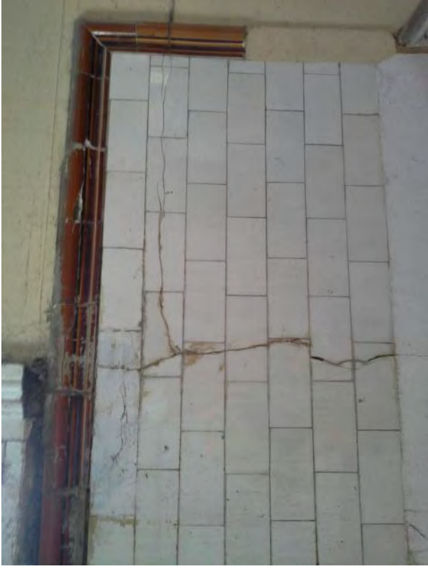
Photograph 12 Typical Cracks to interior walls
