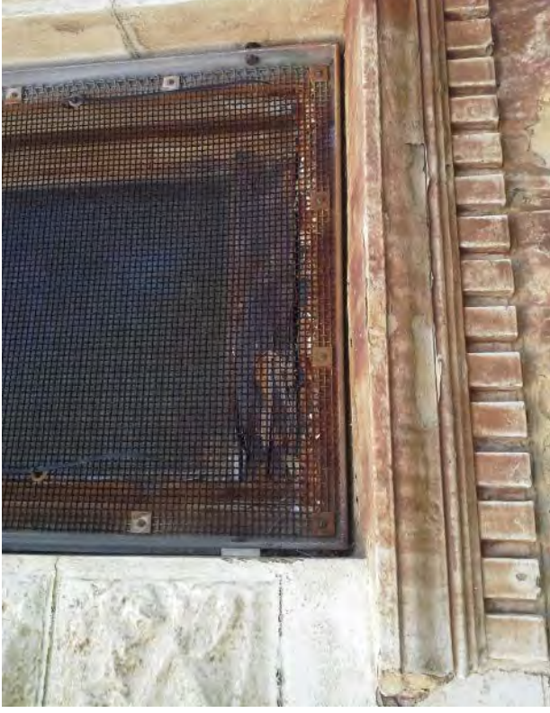
Photograph 11 Deterioration of exterior Window Frame Western End
