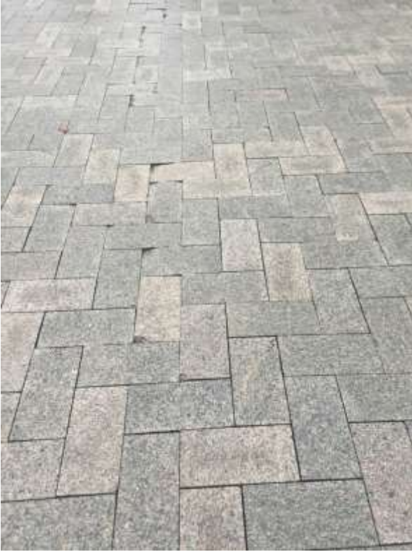
Chipped paver – Trip Hazard
