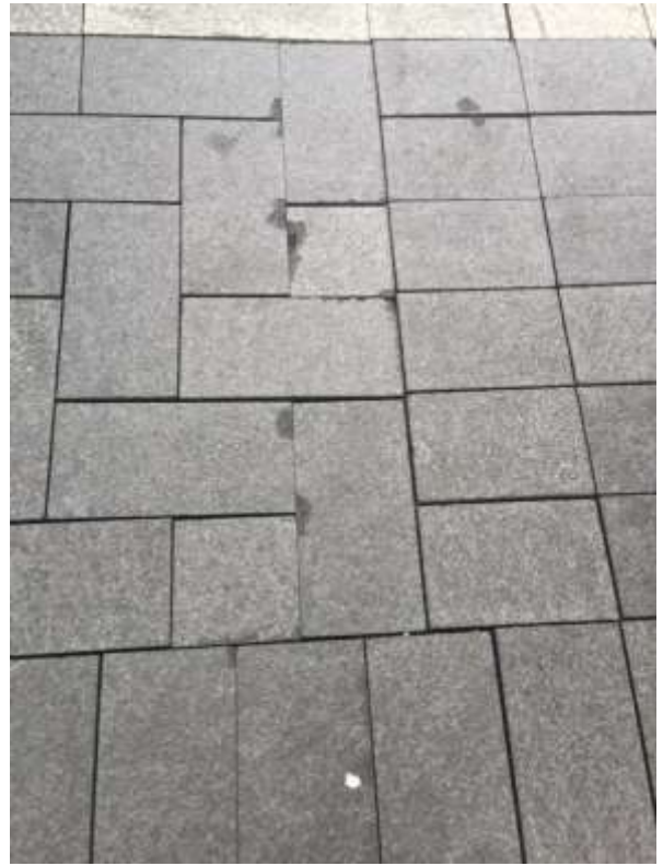
Chipped paver – Trip Hazard
