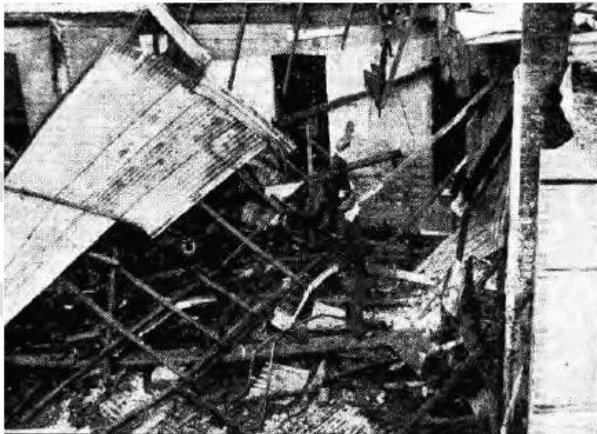
Fire damage in 1950, showing the collapsed roof to Commercial Building, 553 – 561 Wellington Street (The Daily News, 9 October 1950, p. 1)
