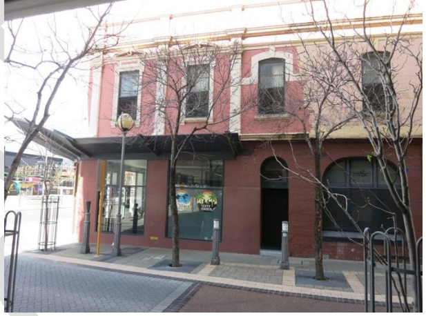
View of Queen Street corner (element, 4 October 2018)
