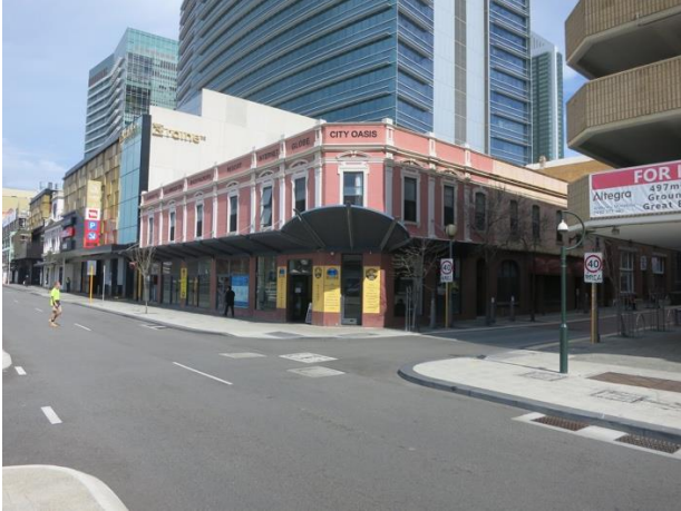
View of corner across Wellington Street (element, 4 October 2018)
