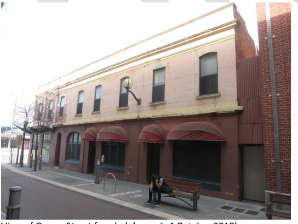
View of Queen Street facade (element, 4 October 2018)
