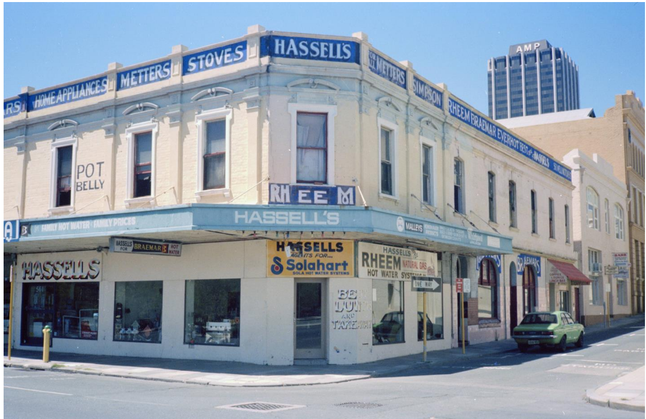
Corner view of Commercial Building, 553 – 561 Wellington Street in 1981 (State Library of Western Australia, ref: slwa_b3800009_1)
