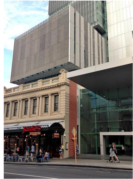
One40william, Corner William and Murray St Mall Street, Perth WA; Architect: HASSELL
