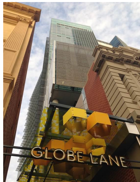
One40william, Corner William and Murray St Mall Street, Perth WA; Architect: HASSELL
