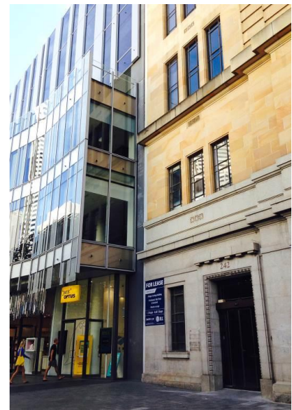
One40william, Corner William and Murray St Mall Street, Perth WA; Architect: HASSELL
