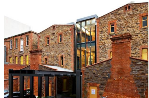
Hayborough Building, Rundle Street, Adelaide, SA; Architect: Tectus
